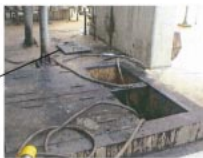
Disposal pit with pit cover removed.
