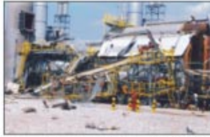
The steam utility boiler after the explosion
