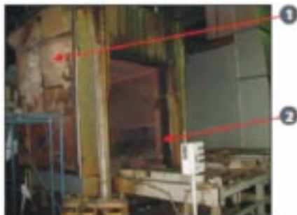
The furnace without its door after the explosion.
